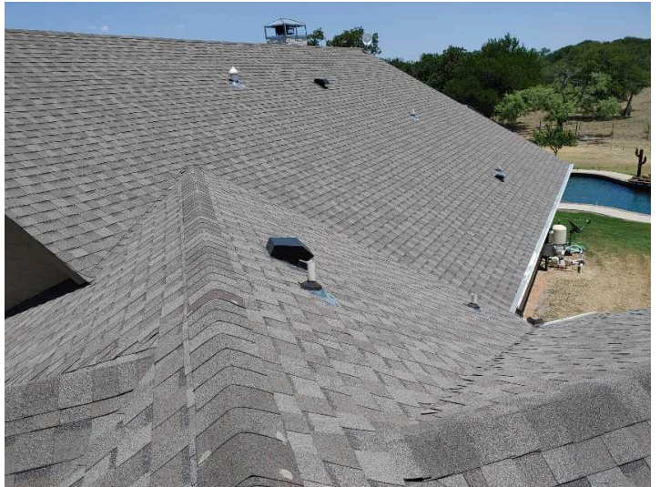
View from West side of roof
