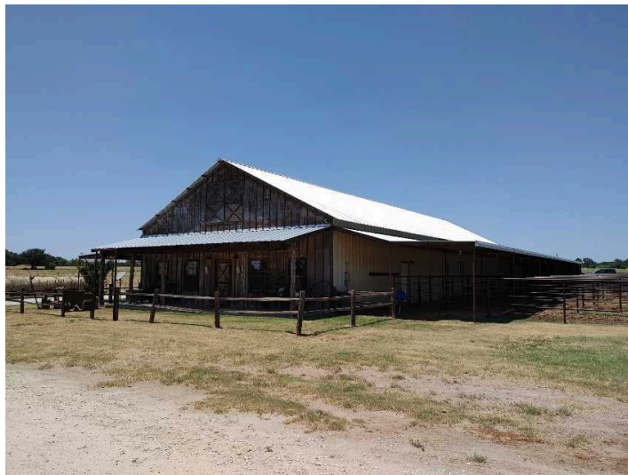
Guest House/Barn/Garage situated North side of property
