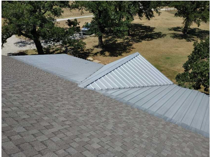
Metal roof covering at front porch appears adequate
