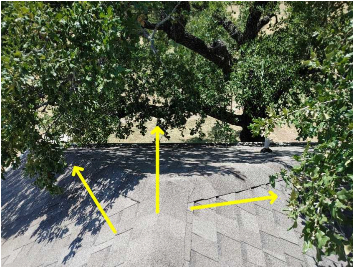
Tree limbs should be trimmed back 6 feet from roofdeck
