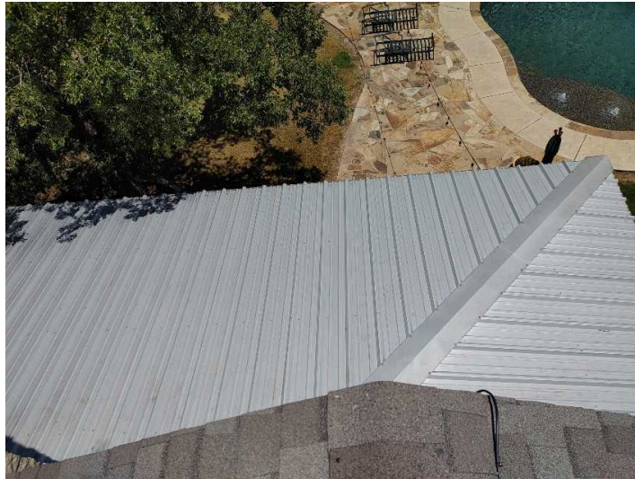
Metal roof covering at side porch appears adequate
