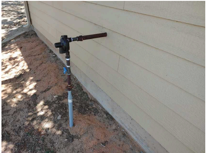
LP gas inlet line to structure appears adequate
