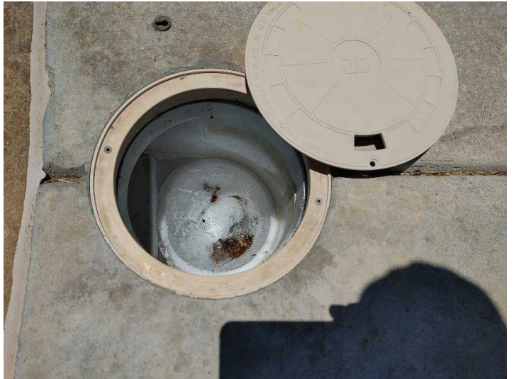
Water level was low at time of inspection
