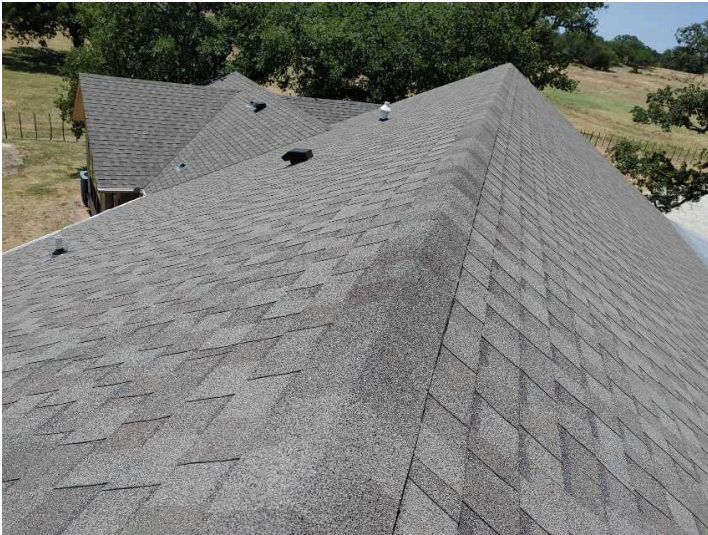
View from East side of roof
