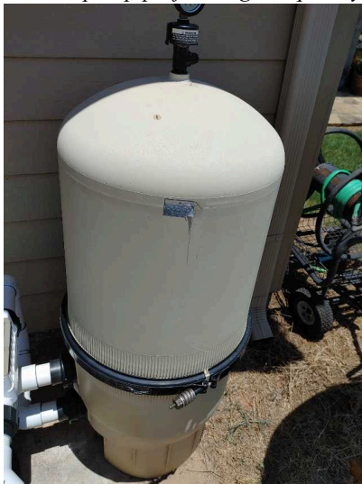
DE Filter tank should be backwashed monthly (Re-add DE after backwashing)
