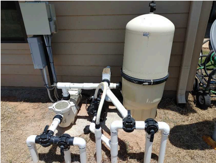
Pool equipment should be protected from UV exposure
