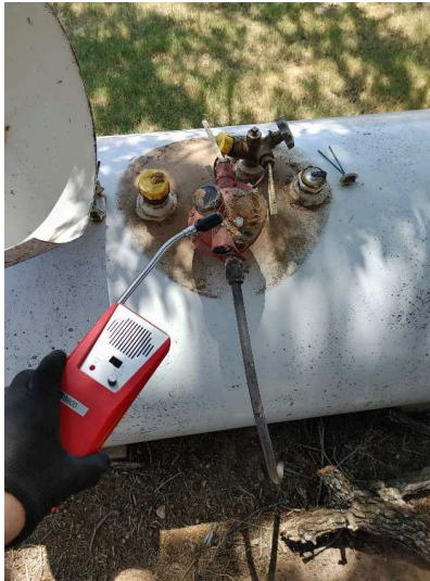
No gas leaks were detected
