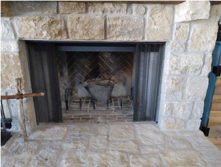
Glass cover should also be applied to front of firebox for additional protection from fire hazards
