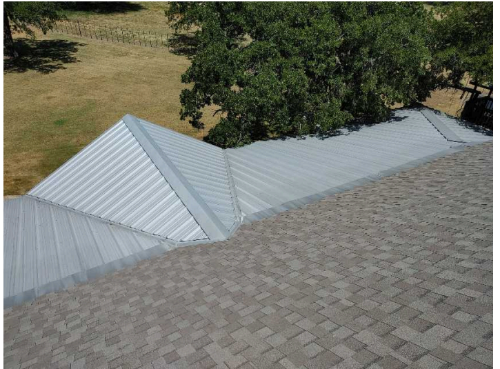
Metal-tin roof located over porch coverings (Adequate)
